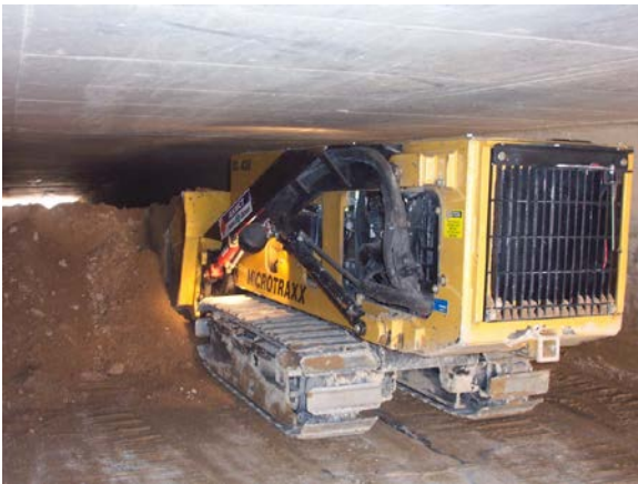
Figure 1- Tunnel mucker in 4 ft high box culvert.
