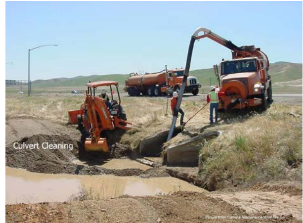
Figure 4 - Culvert cleaning with a vacuum truck.
