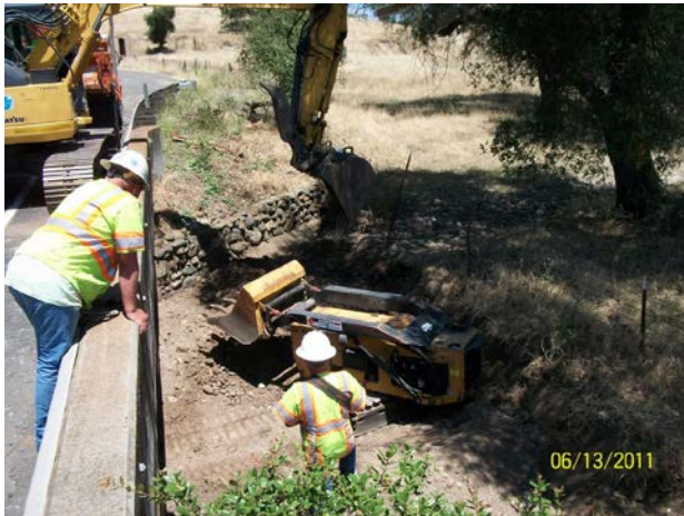
Figure 2- Tunnel mucker at job site with excavator.
