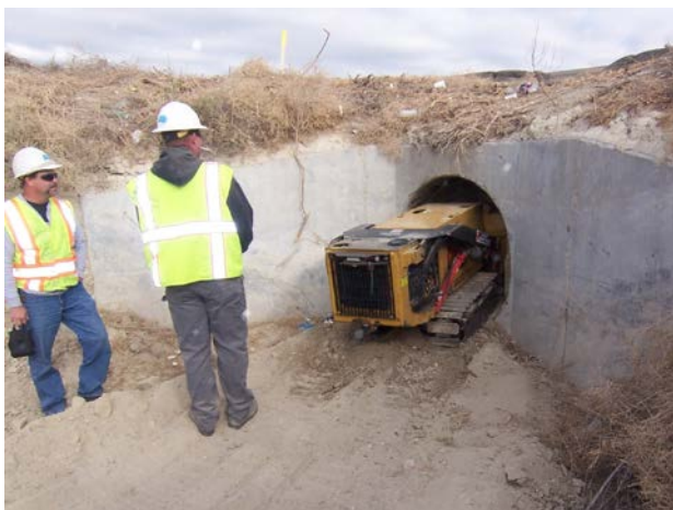
Figure 3- Tunnel mucker in 5 ft round culvert.
