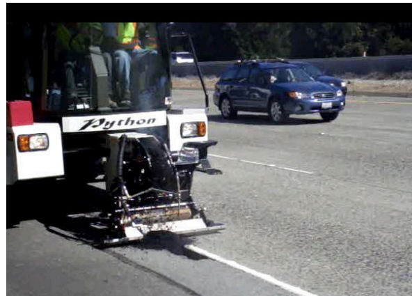
Python Automated Hot Asphalt Patching
