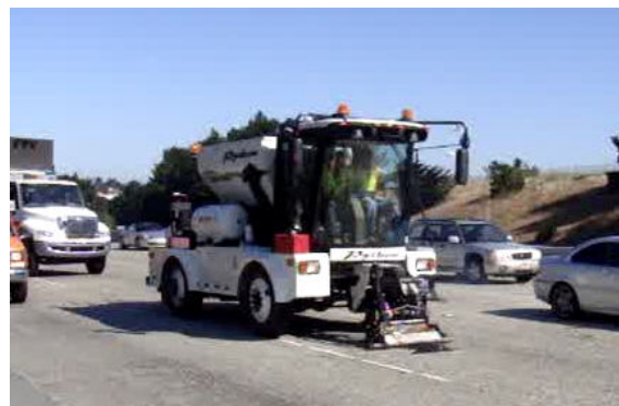
Python Rolling Patching Operation – Interstate 280
