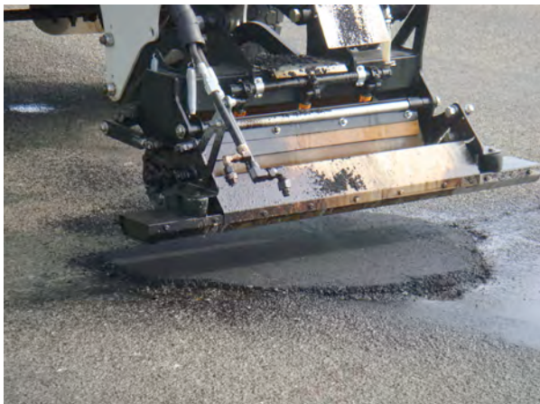
Figure 1 – Python hot asphalt pothole patch
