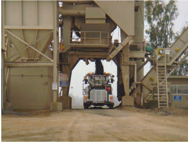
Figure 3 – Loading Python with Hot Asphalt
