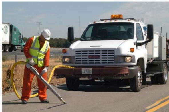
Figure 2 – Sealzall, In-Lane Sealing Configuration
