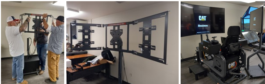
Figure 4.4: Left and middle: Installation of Caterpillar screen stand; installed Caterpillar simulator
