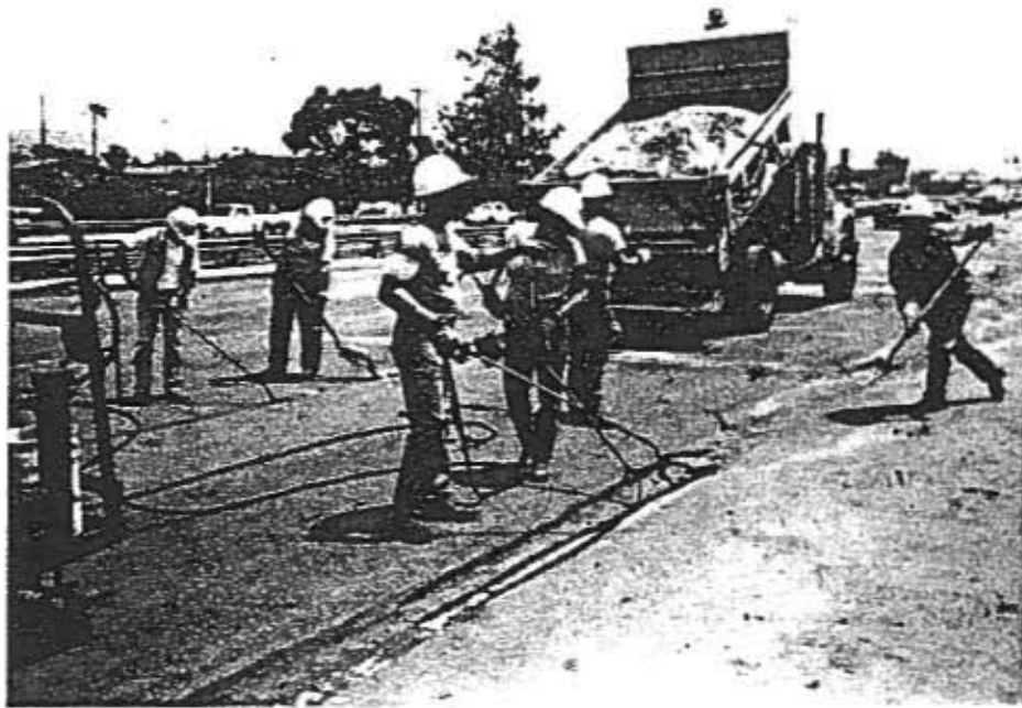
FIG. 9: LONGITUDINAL AND TRANSVERSE CRACK FILLING
