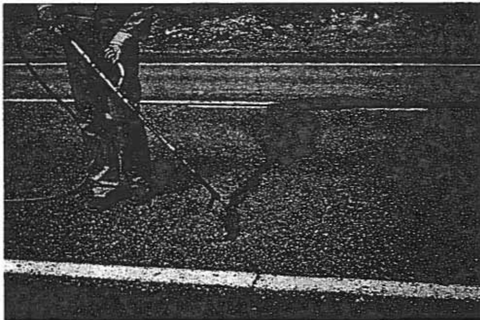
FIG. 10: TRANSVERSE CRACK FILLING WITH CRS-2 AND SAND BLOTTER
