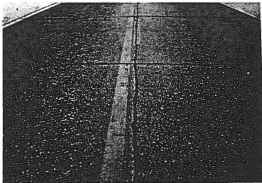
FIG.8: CRACK AND JOINT REPAIR ACCOMPLISHED WITHOUT SQUEEGEE
