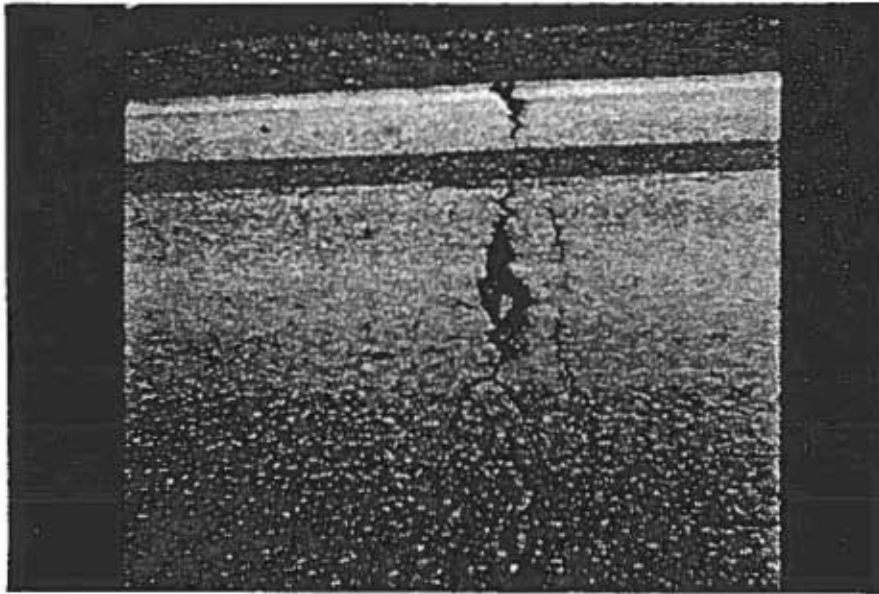
FIG. 14: JOINT DETERIORATION DUE TO MOISTURE
