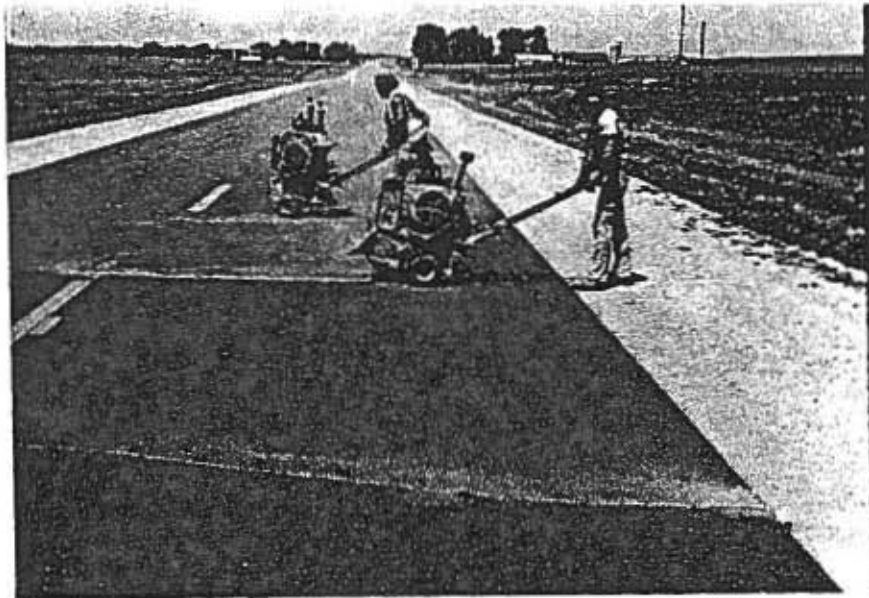
FIG. 5: ROUTING OF TRANSVERSE CRACKS
