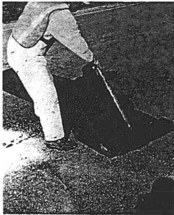
FIG. 15: USING LUTE TO SPREAD SLURRY
