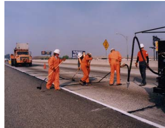
Hand Operation Sealing All Cracks
