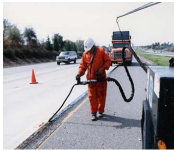
Longitudinal Sealing by Hand
