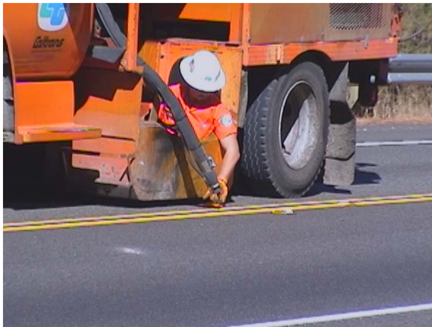
Figure 2: The traditional RPM placement action
