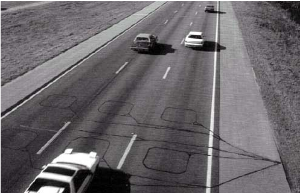
Figure 2.1: Traffic detector, double inductive loop [5]
