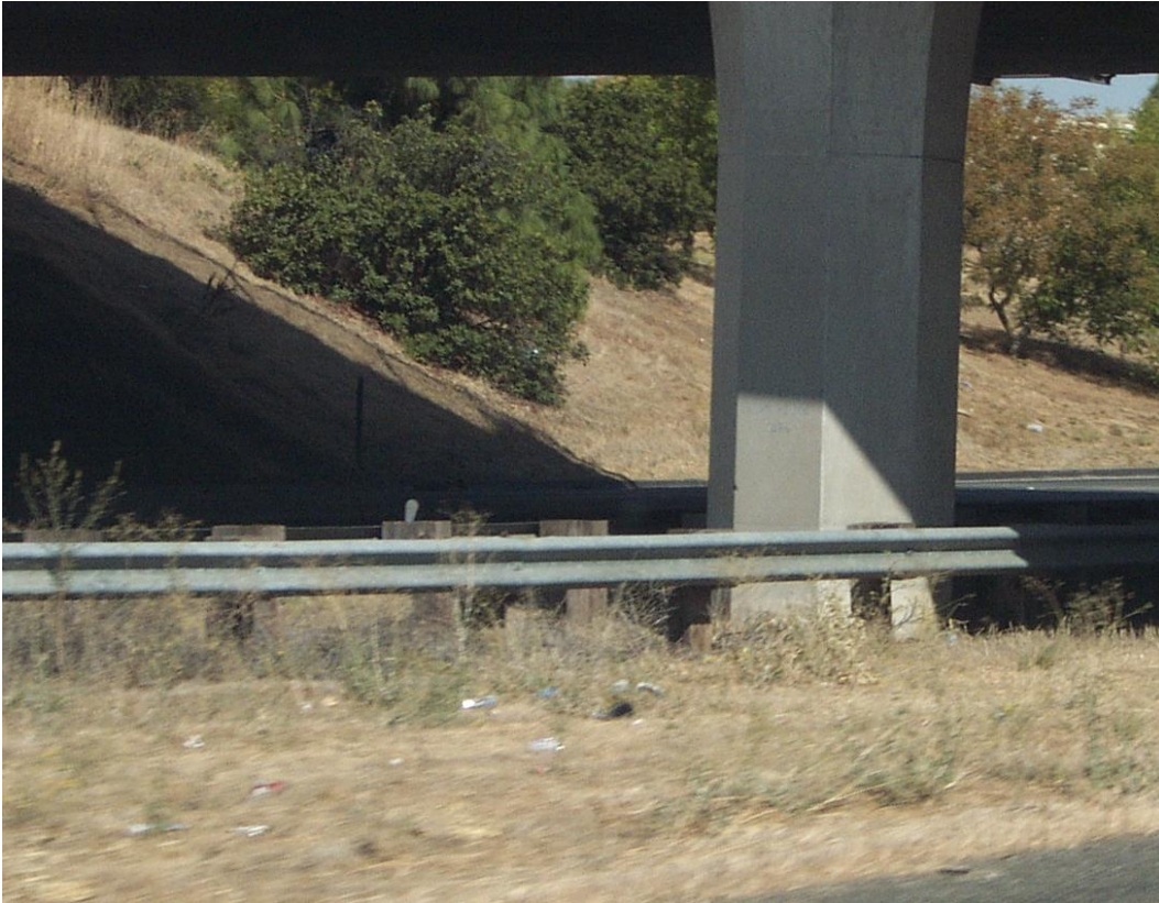
Figure 2.1 Guardrail Around Overpass Support
