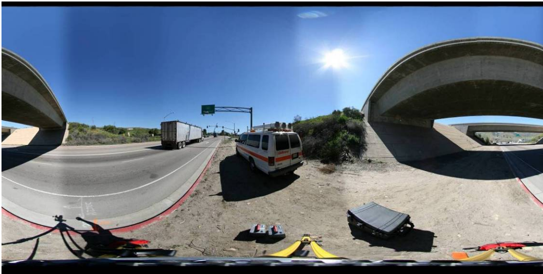
Figure 11: Example panoramic photograph, District 11, Mast Boulevard at Highway 52
