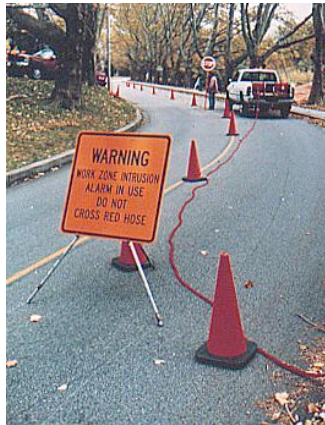
Figure 2. Typical Perimeter System Using Pneumatic Tubes [3]
