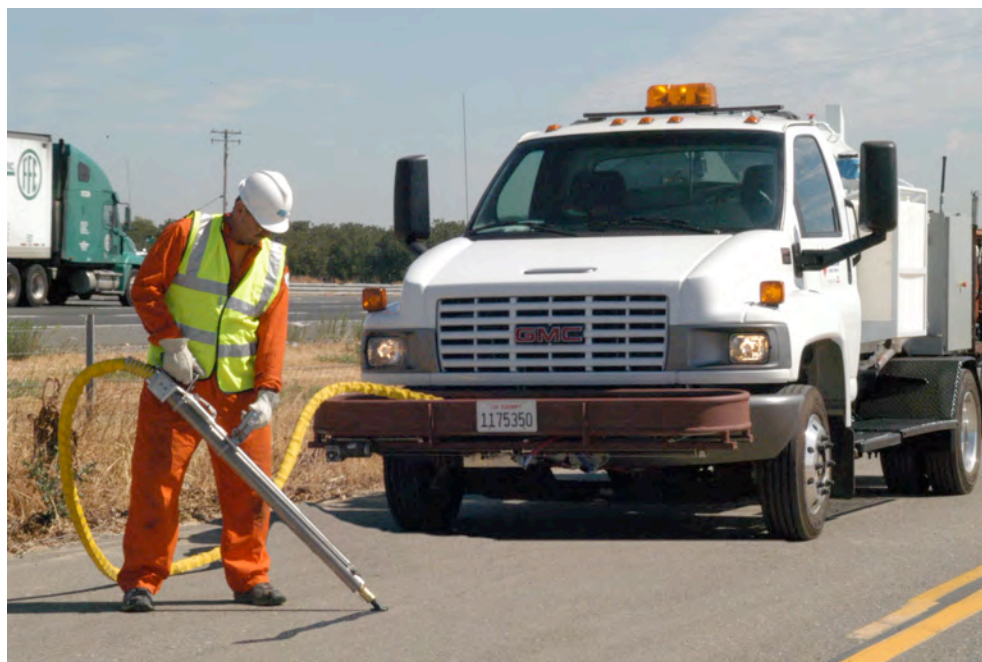
Figure 11. Sealzall In-Lane Sealing
