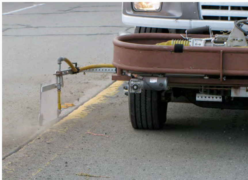
Figure 8. Longitudinal Crack Cleaning
