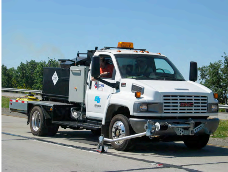
Figure 5. TTLS Appl. Truck Sealing Hwy 113
