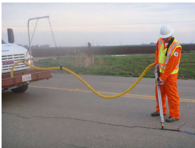
Figure 37. Manual Sealing Hose and Support Boom
