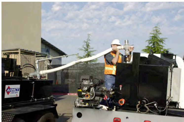
Figure 3. TTLS Sealant Transfer
