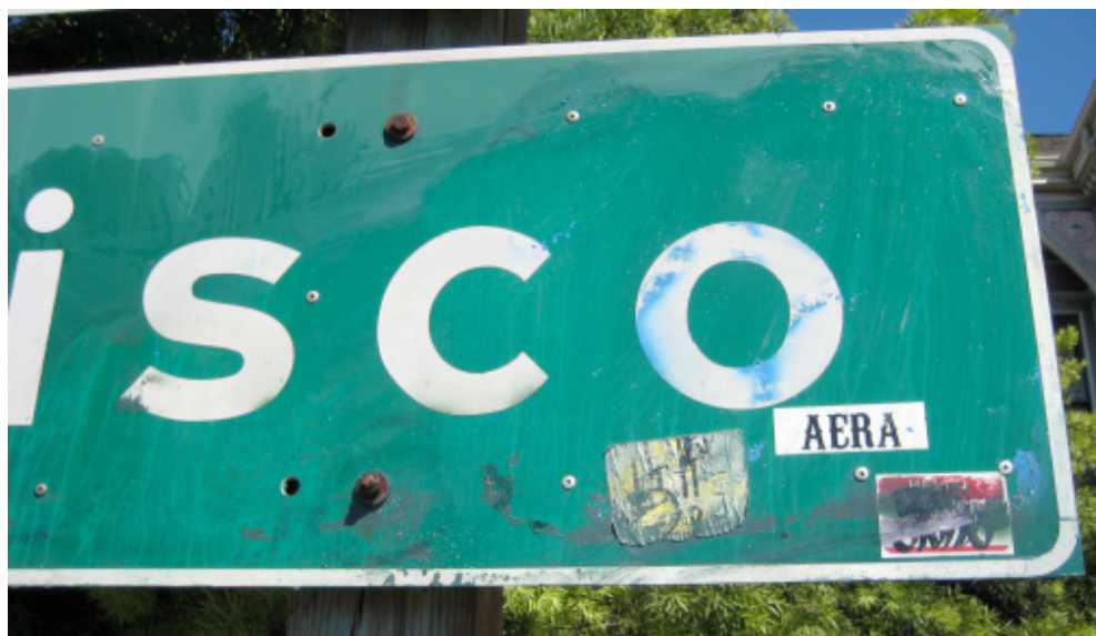
Figure 1-7: Older sign with non-reflective decals
