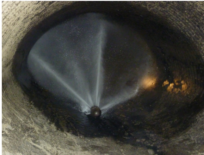
Figure 2.8: Sewer jet flushing debris in a culvert
