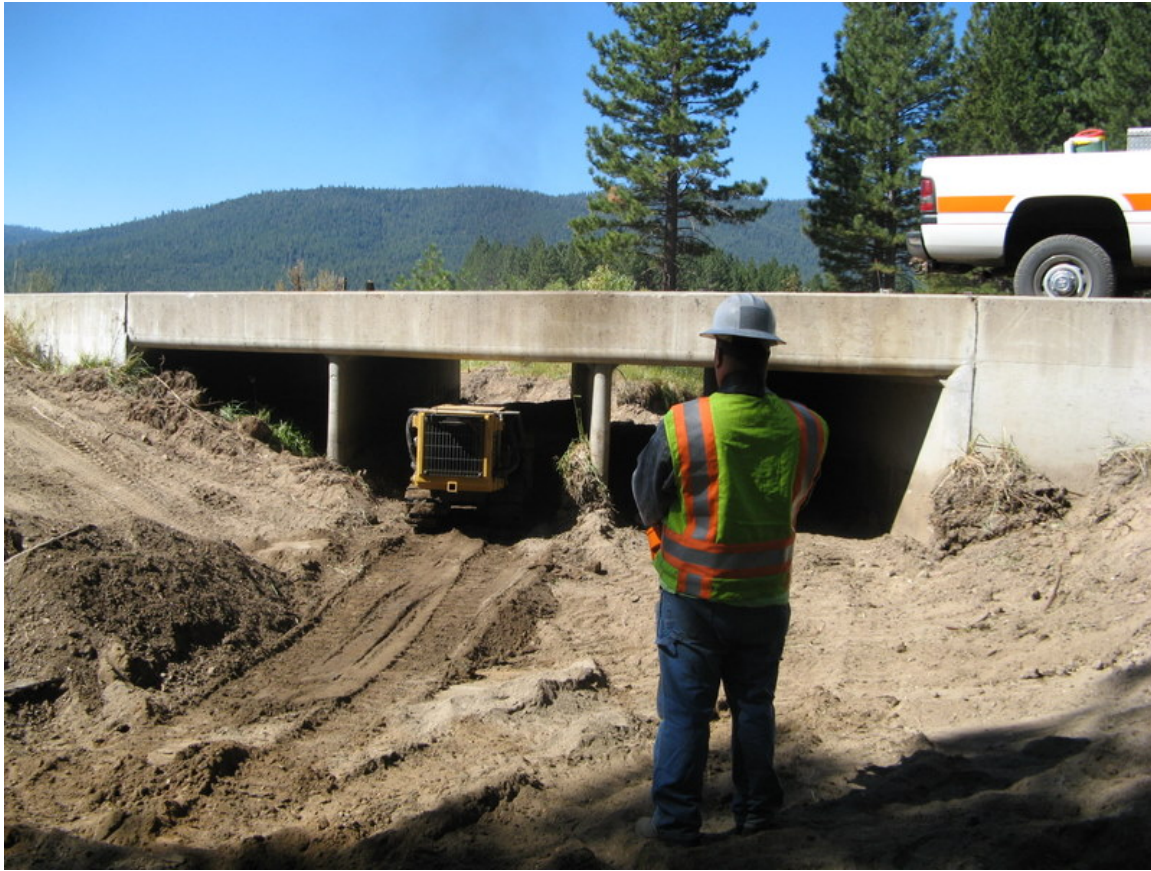
Figure 3.2: Mucker enters to collect a bucket full
