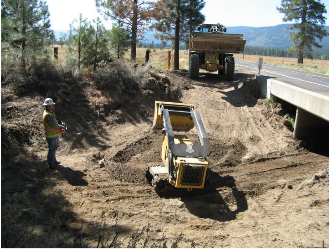
Figure 3.3: Slews to dumps material at the base of ramp
