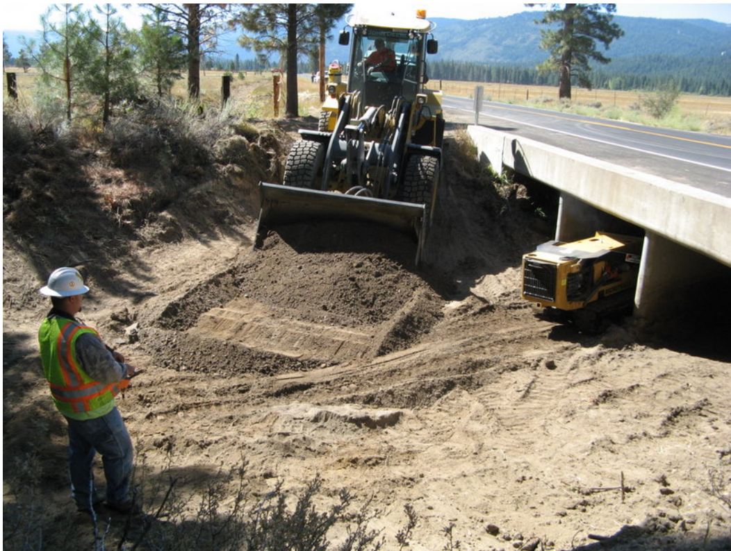
Figure 3.4: Loader moves debris from mucker staging area to dump truck
