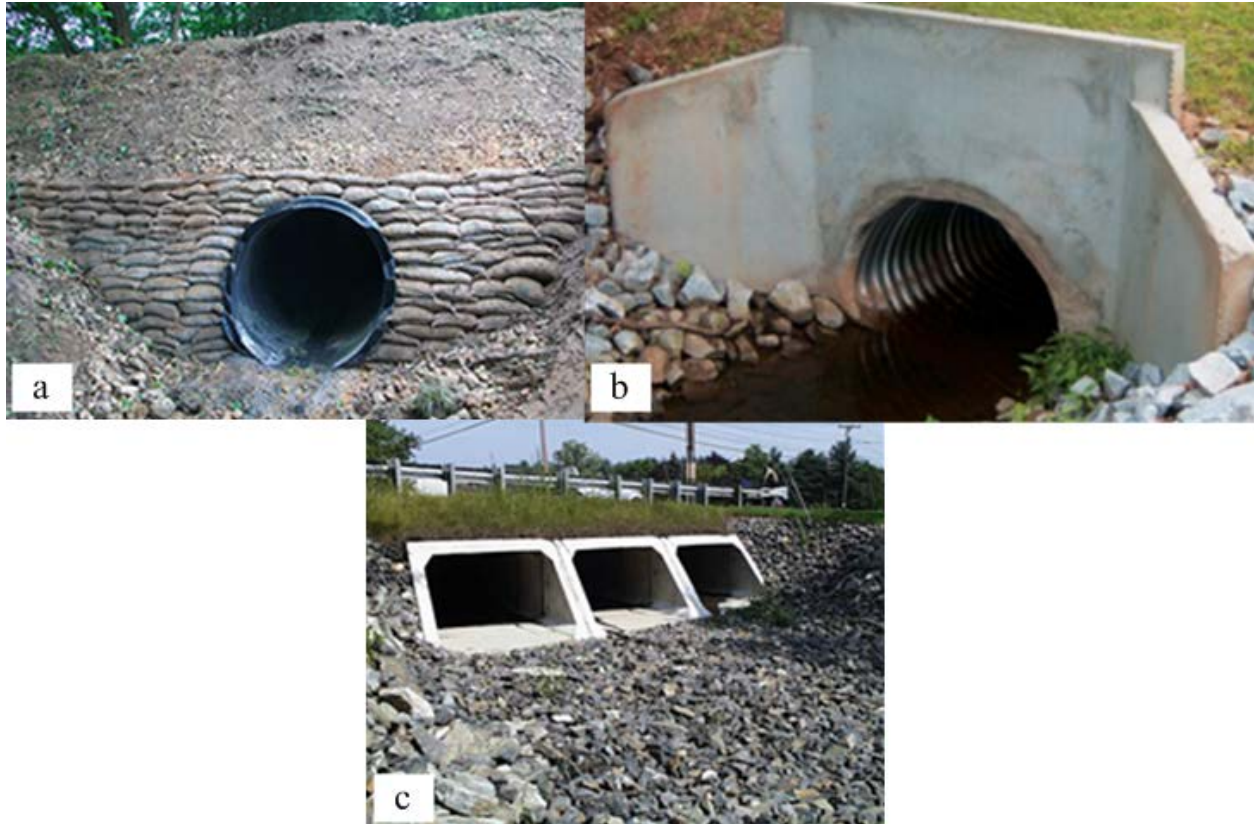
Figure 2.2: (a) Headwall constructed with hessian sacks filled with semi-dry C20 concrete mix [6] (b) Concrete headwall with two wingwalls [7] (c) Triple concrete box culvert [8]
