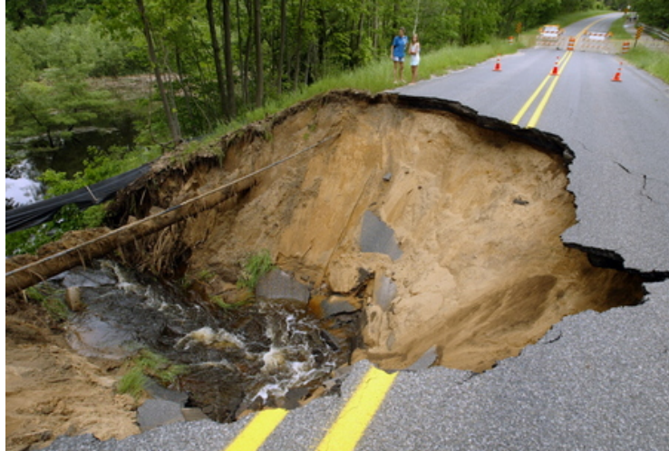
Figure 2.6: Highway washout due to culvert failure [11]
