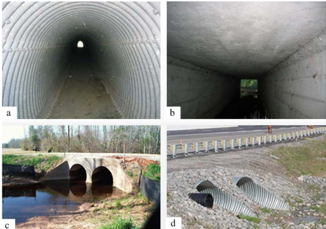
Figure 2.1: (a) Corrugated steel pipe [3] (b) Concrete box culvert [3] (c) Concrete culvert for stream crossing [2] (d) Corrugated steel pipe culvert [4]
