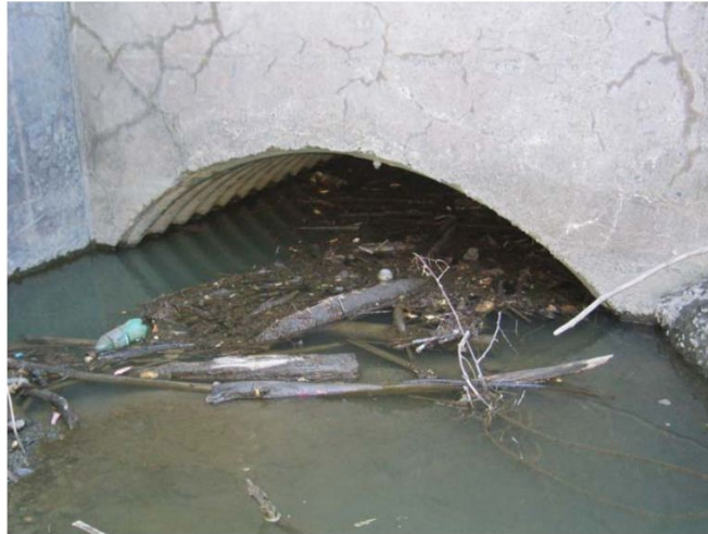
Figure 2.4: Blocked culvert [3]
