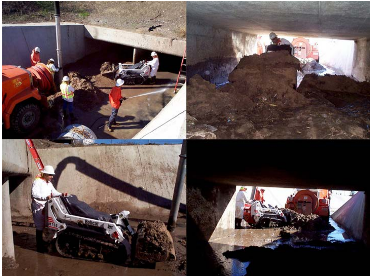
Figure 2.10: Using a walk-behind loader to clean the culvert
