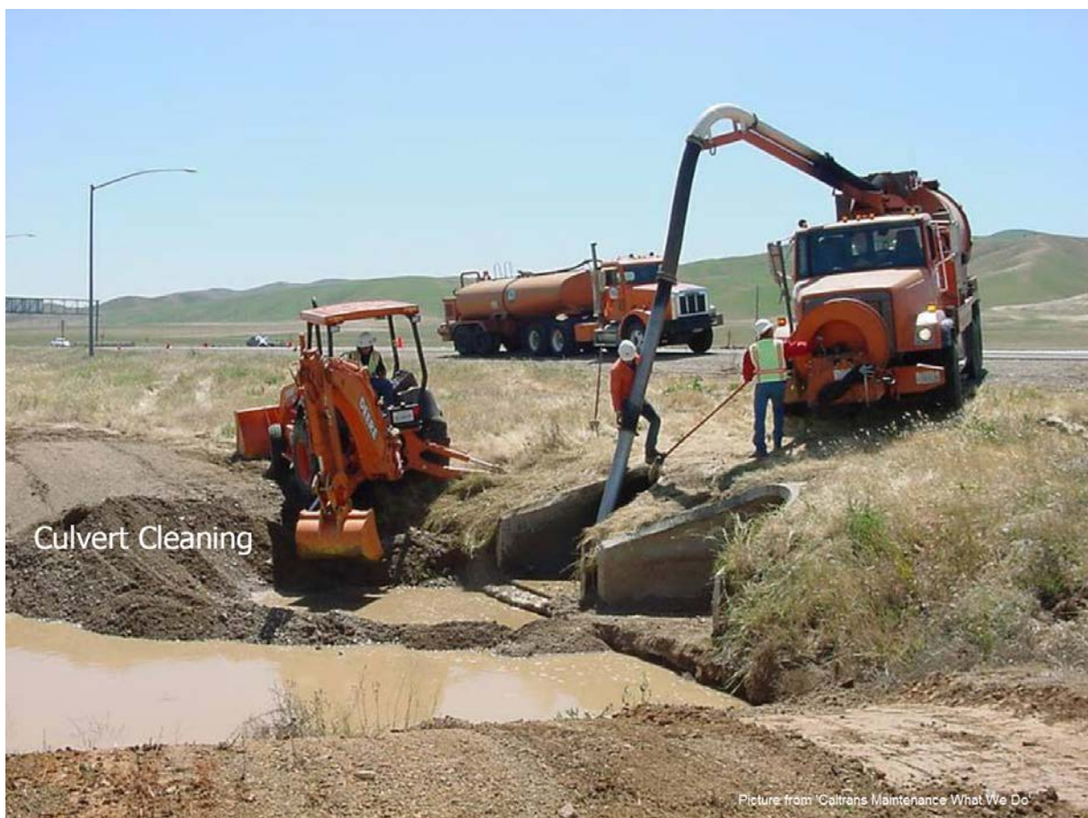
Figure 2.7: Vacuum truck culvert clearing operation (From Caltrans Maintenance What We Do)
