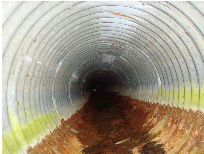
Figure 2.3: Rusty corrugated culvert [9]
