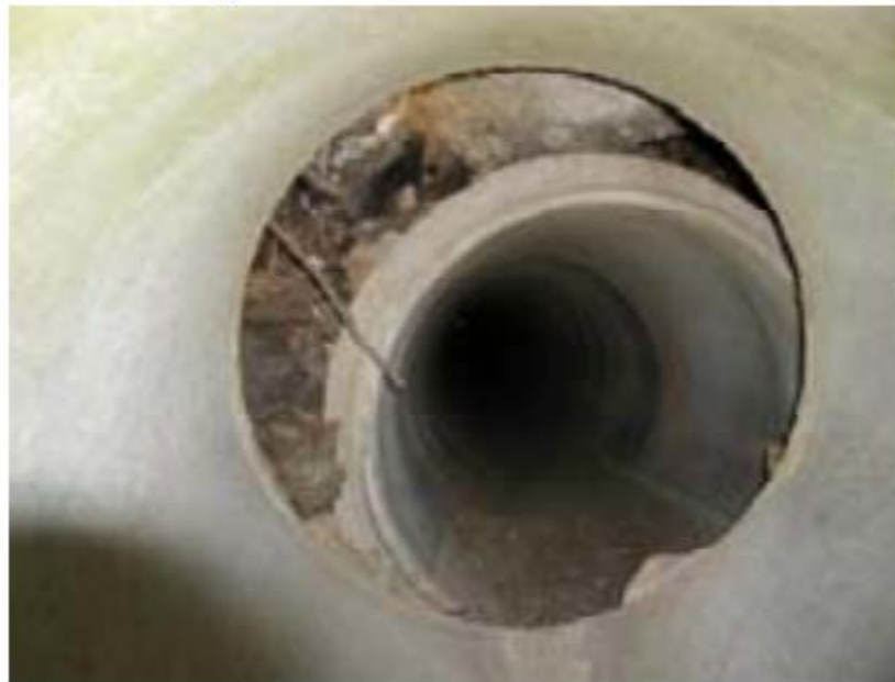
Figure 2.5: Joint failure in a round concrete culvert [10]
