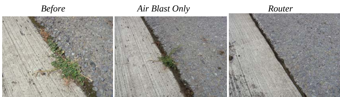
Figure 15. Crack Cleaning Test - Interstate 380
