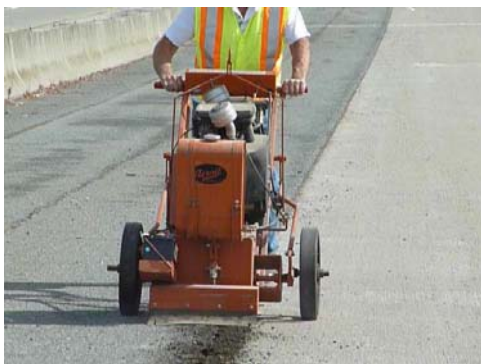
Figure 17. Joint Routing - Interstate 380
