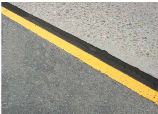
Figure 13. Effective Joint Seal - Hwy 160
