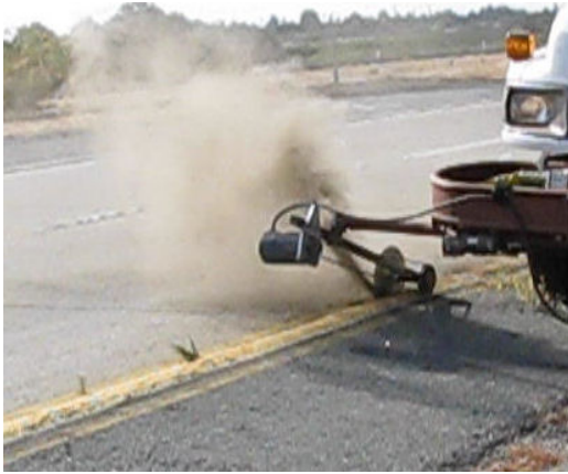
Figure 16. Sealzall Crack Cleaning Attachments – Hwy 160
