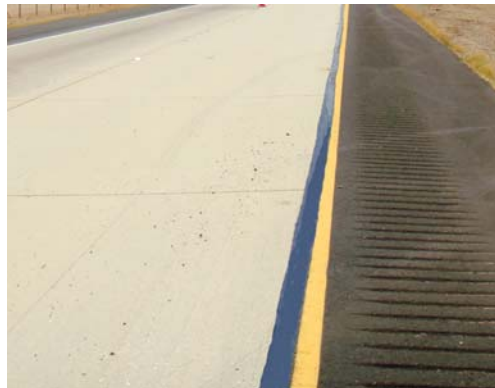
Figure 14. Effective Joint Seal - Interstate 8
