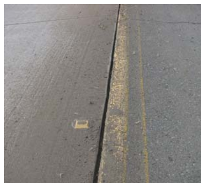
Figure 22. One Pass Routed Joint
