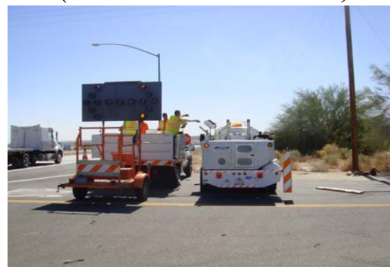
Figure 5. Loading Sealant Blocks - Hwy 86
