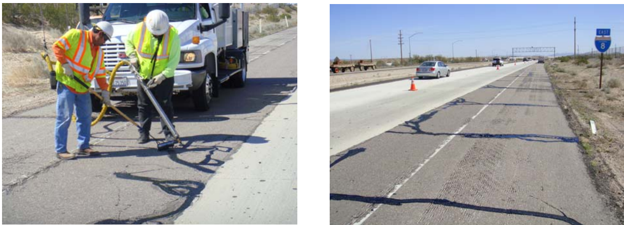
Figure 6. Merge Lane Manual Sealing - Hwy 8
