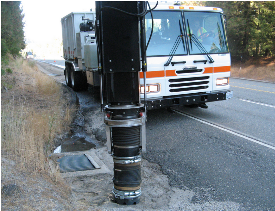
Figure 5.4 - Using the nozzle rotation to break up sand
