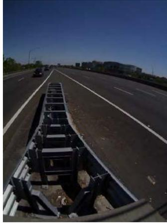
**Figure 12 Daytime view of Smart Cushion installation**
