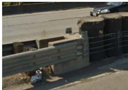
**Figure 2: Backside of REACT 350 attenuator.**
