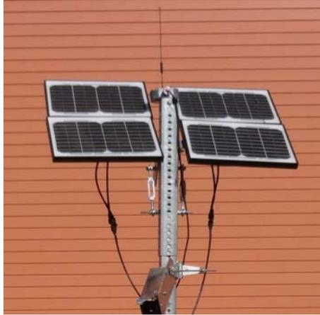
**Figure 121 Mounted solar panel arrangement (ALEK0® 10W Monocrystalline solar panel).**
