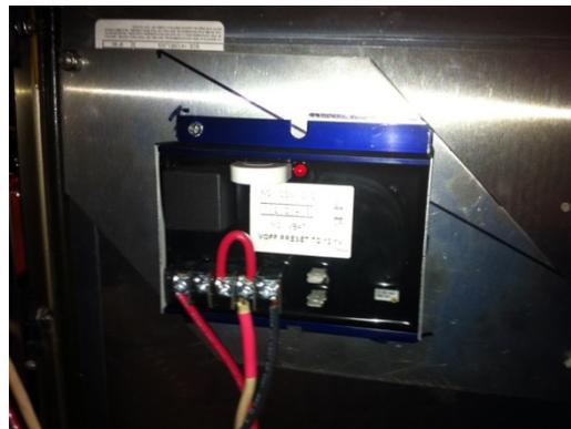
Figure 73: Physical Mounting for Low Voltage Disconnect.
