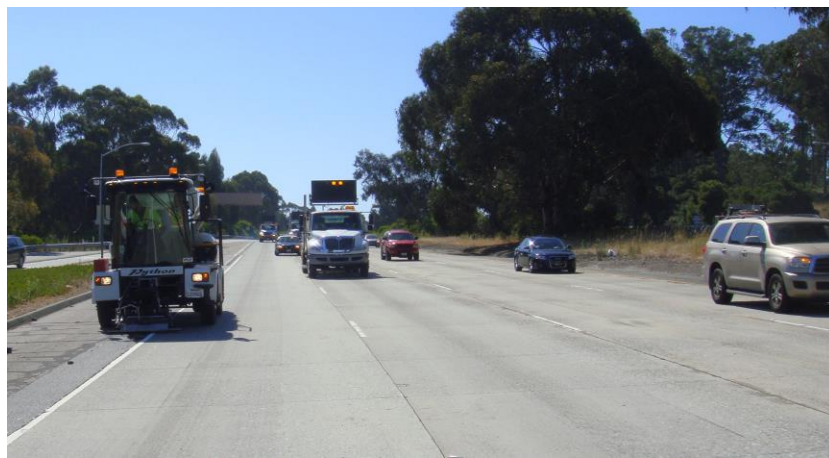
Figure 4. Caltrans Moving Closure Patching Operation
