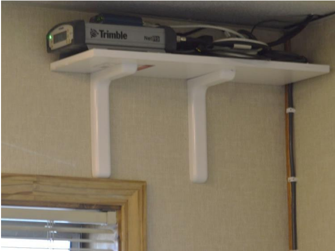
Figure 2.16: GNSS base station receiver and mobile network modem installation at Kingvale Command Center
