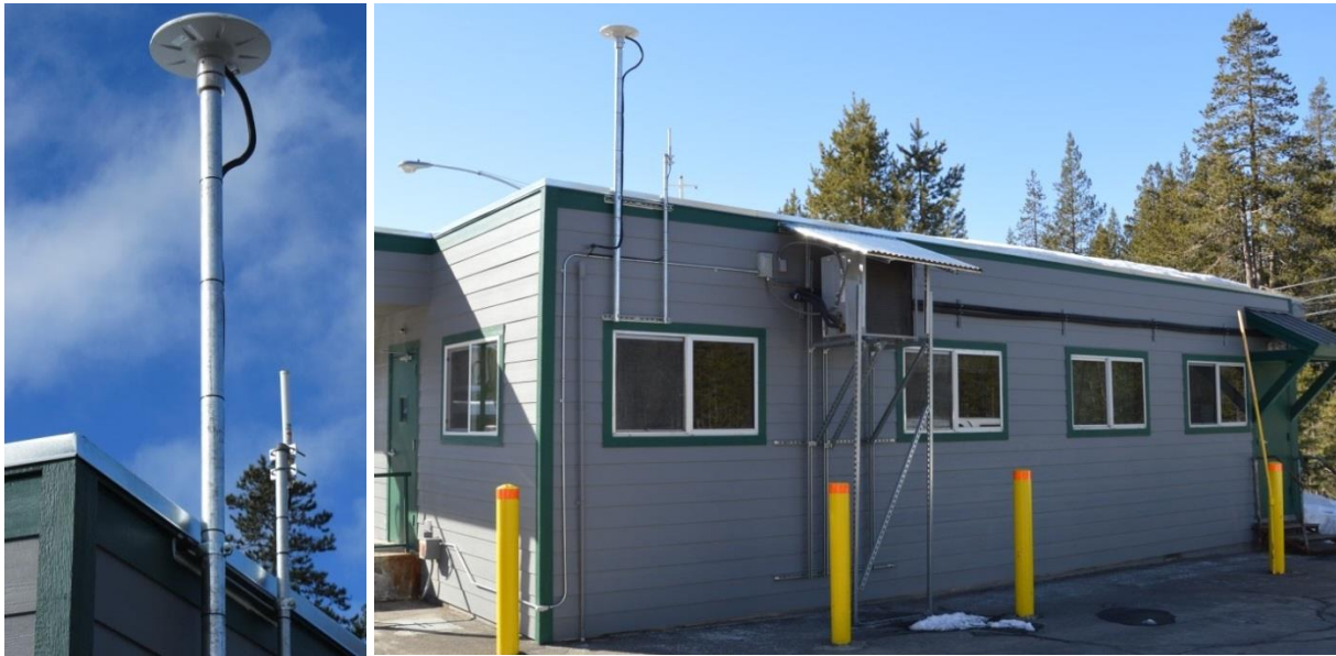
Figure 2.15: GNSS base station antenna and mobile network antenna installation at Kingvale Command Center
