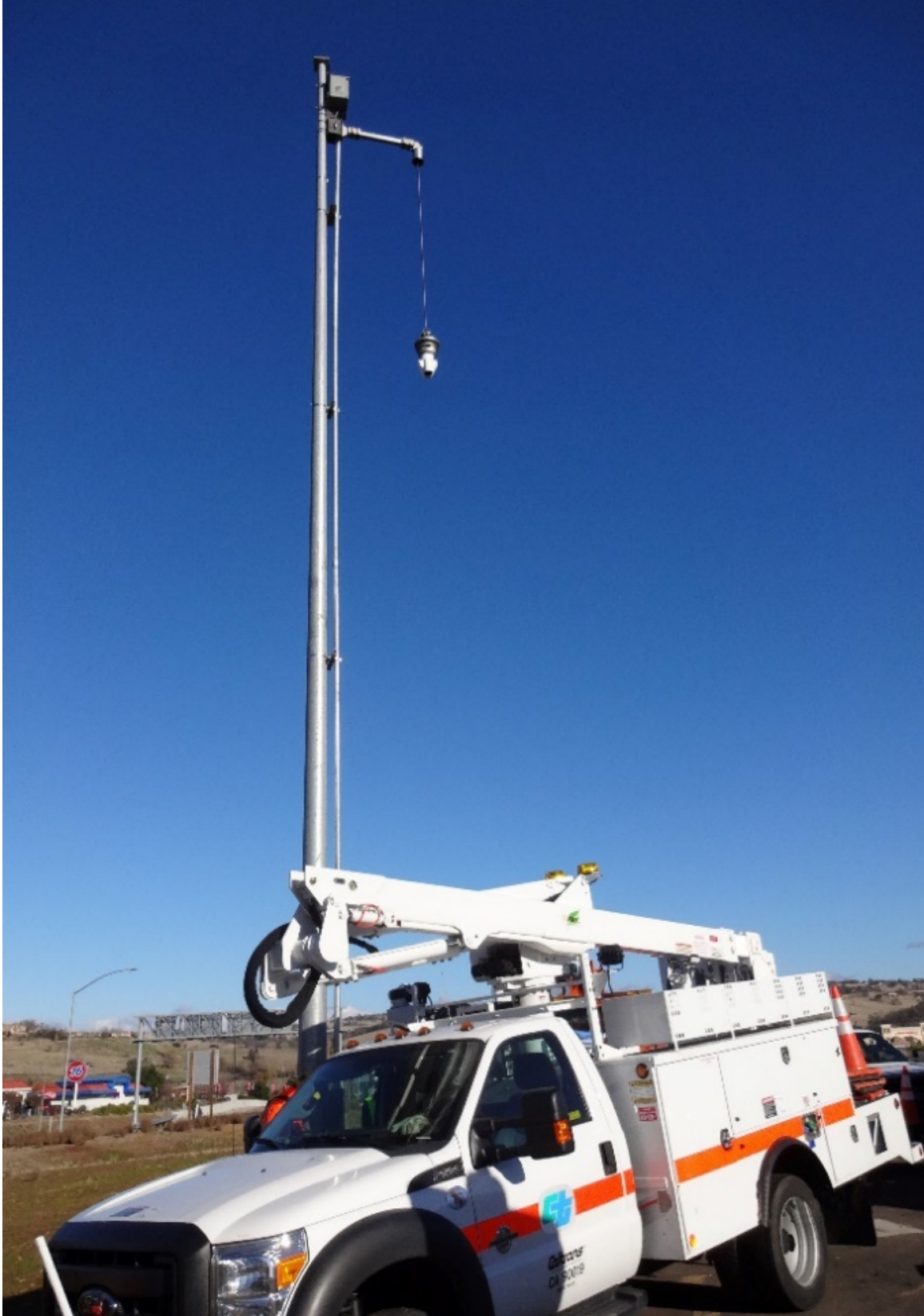
Figure 46. Lowering CCTV Camera MG2 External-Type CLD
