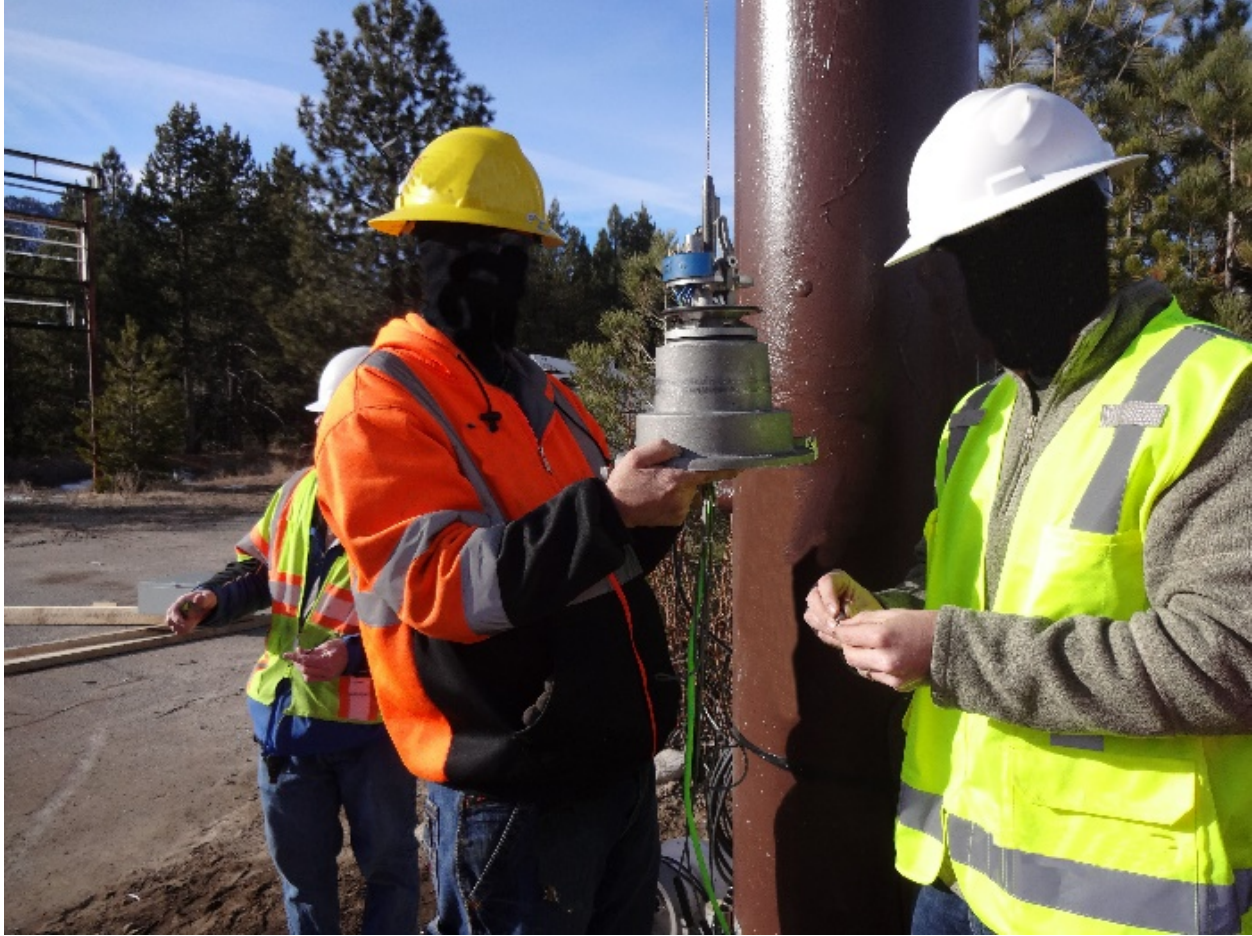
Figure 36. Attaching Coupling Junction Box
