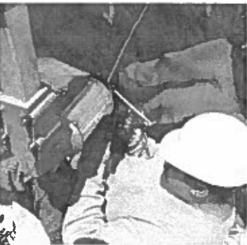
Keeping slight tension on the Lowering cable, engage the bottom contact and perform a continuity check
