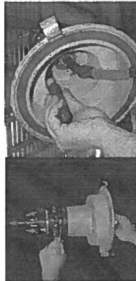
Lower Bottom Contact Unit, using Pull Cord as necessary
