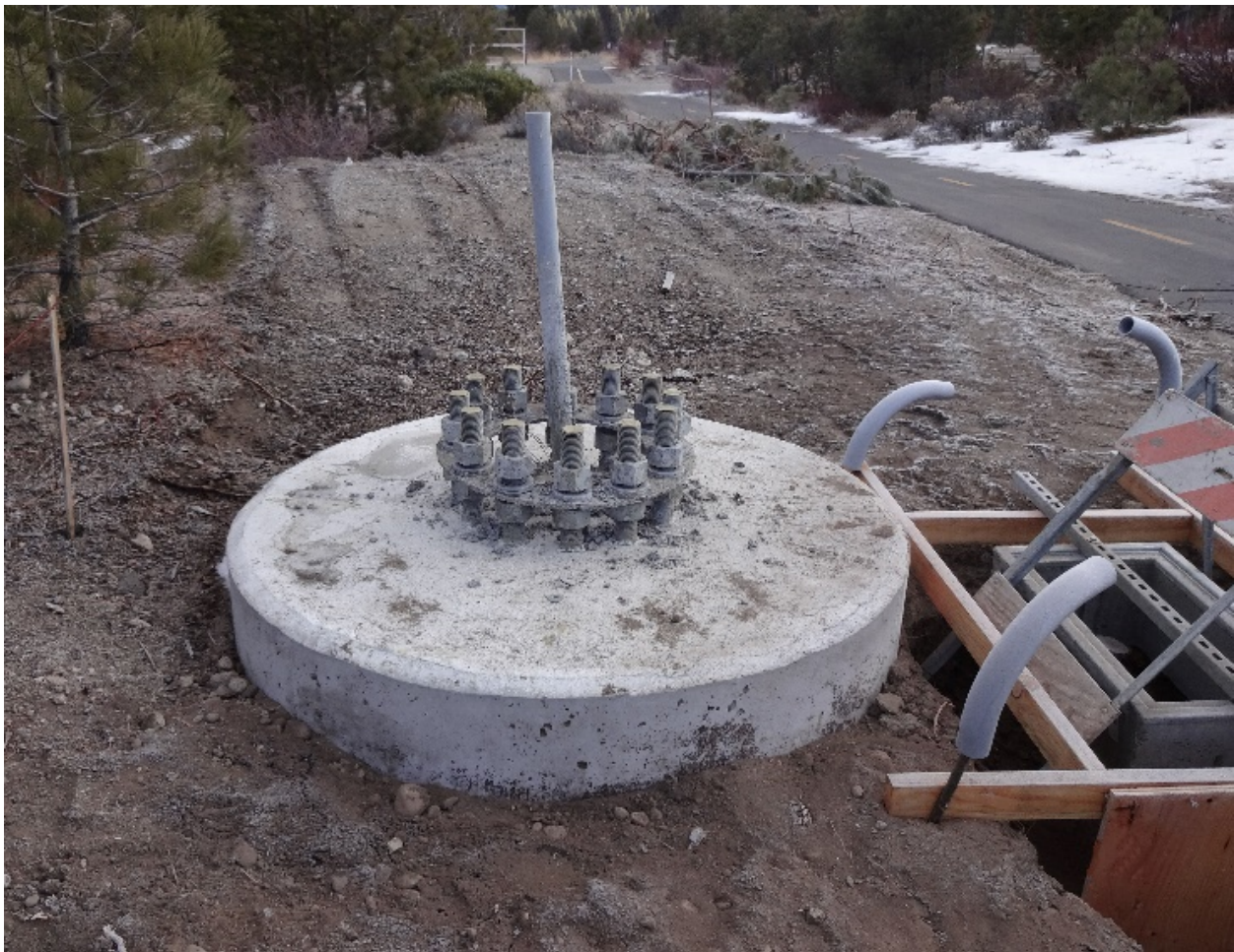
Figure 28. MG 2 Internal-type CLD Pole Footing
