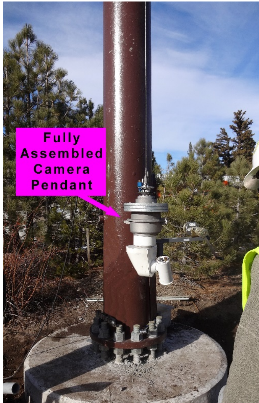
Figure 38. Fully-Assembled Camera, Pendant Lowered
