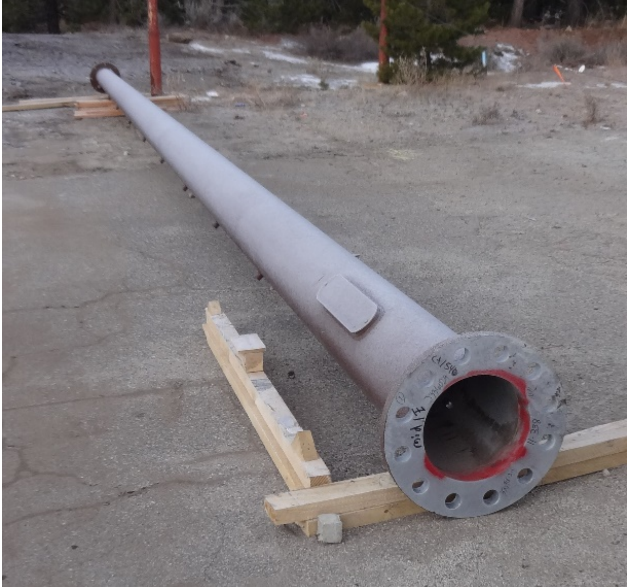
Figure 26. MG 2 Internal-Type Mounted Pole
