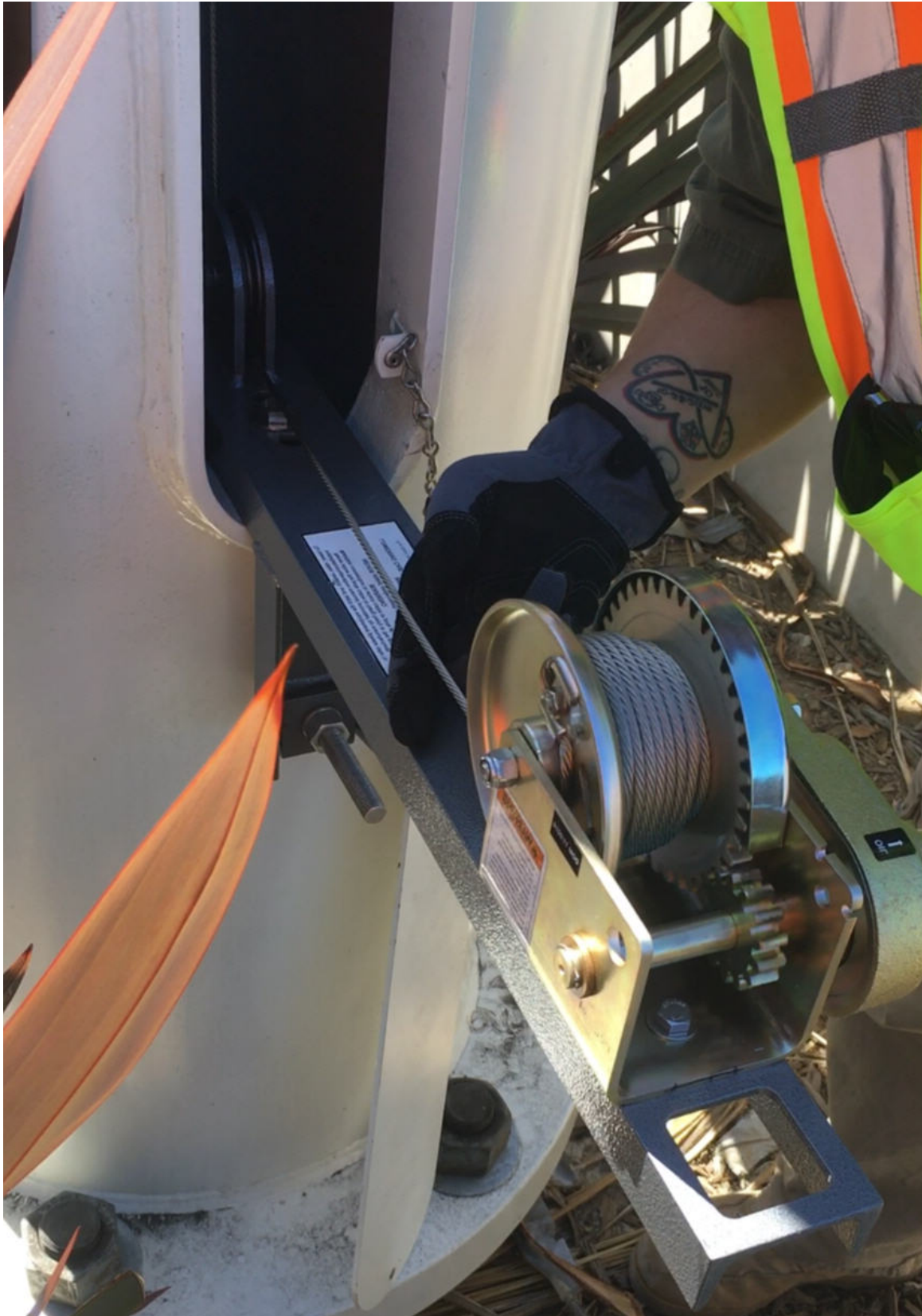
Figure 63. Hand Guiding Winch Cable
