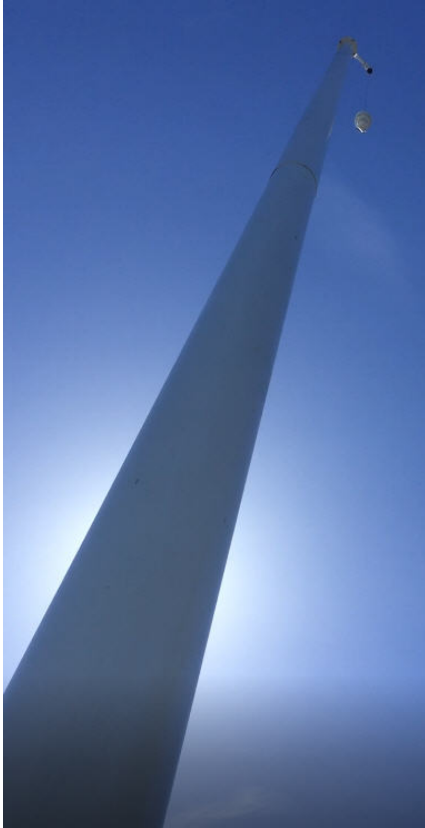
Figure 20. Bay Bridge High-Mast MG 2 Internal-Type CLD System
