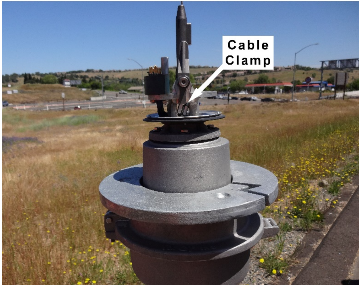
Figure 43. MG 2 External-Type CLD Cable Clamp
