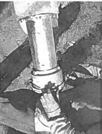
Secure the Pole-Top Junction Box and cover.
