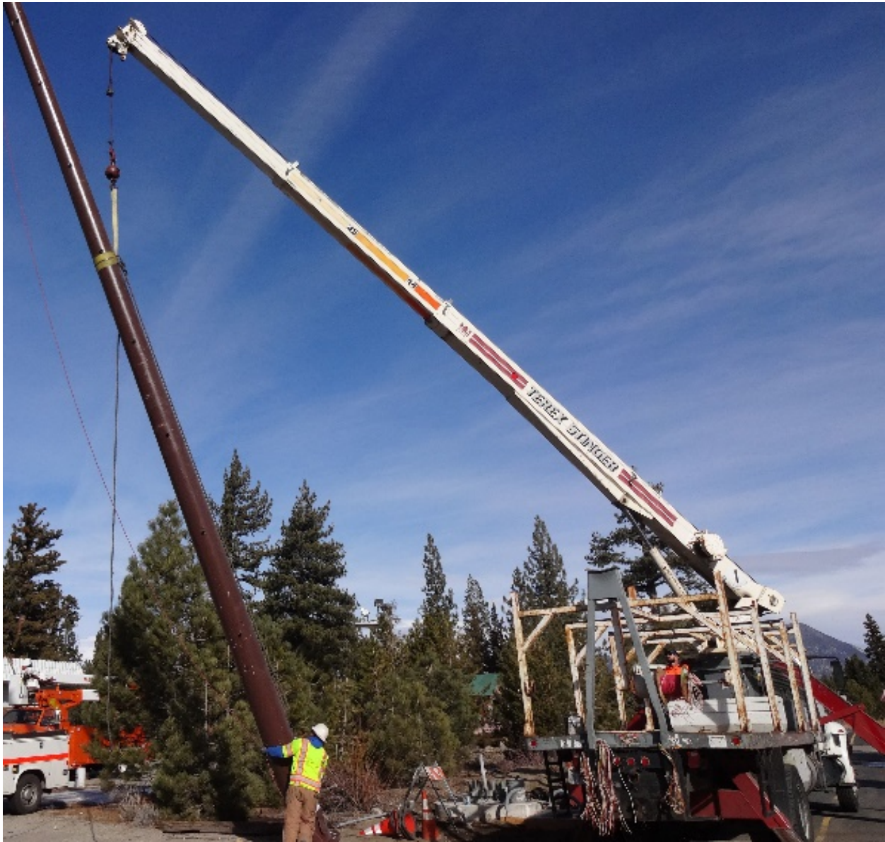
Figure 29. Crane Truck Erecting Pole
