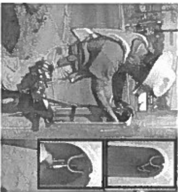
Attach Winch to Pole
