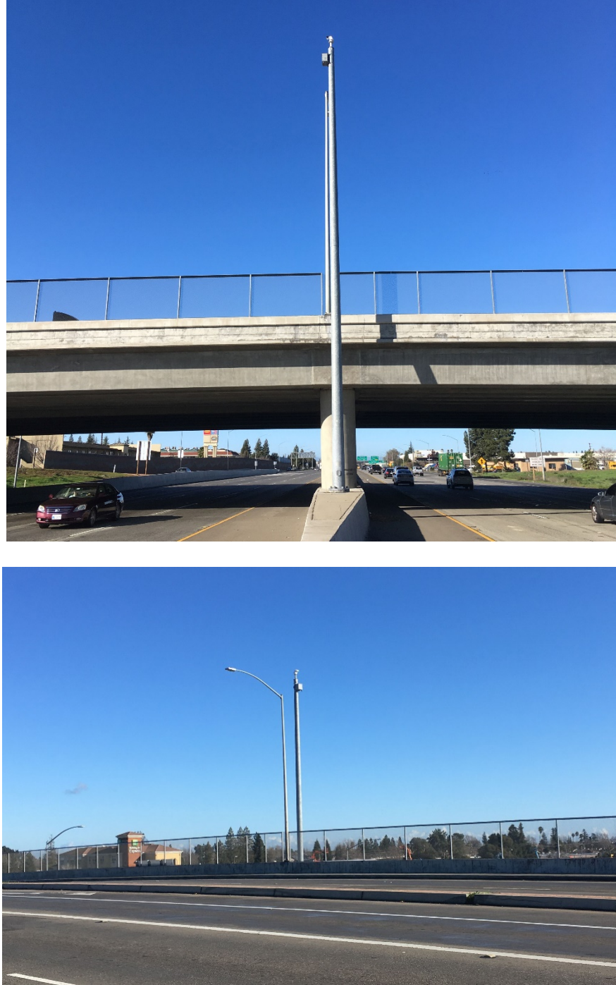
Figure 1. High-Mast Fixed Camera Mounting with Overpass Access
