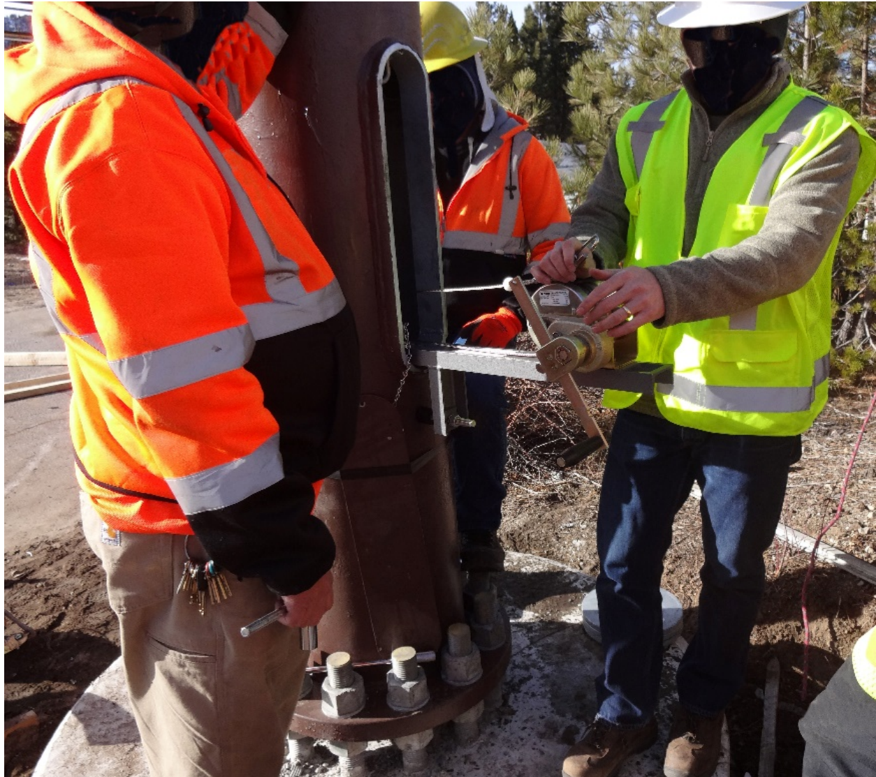
Figure 34. MG 2 CLD Winch Tool Attached
