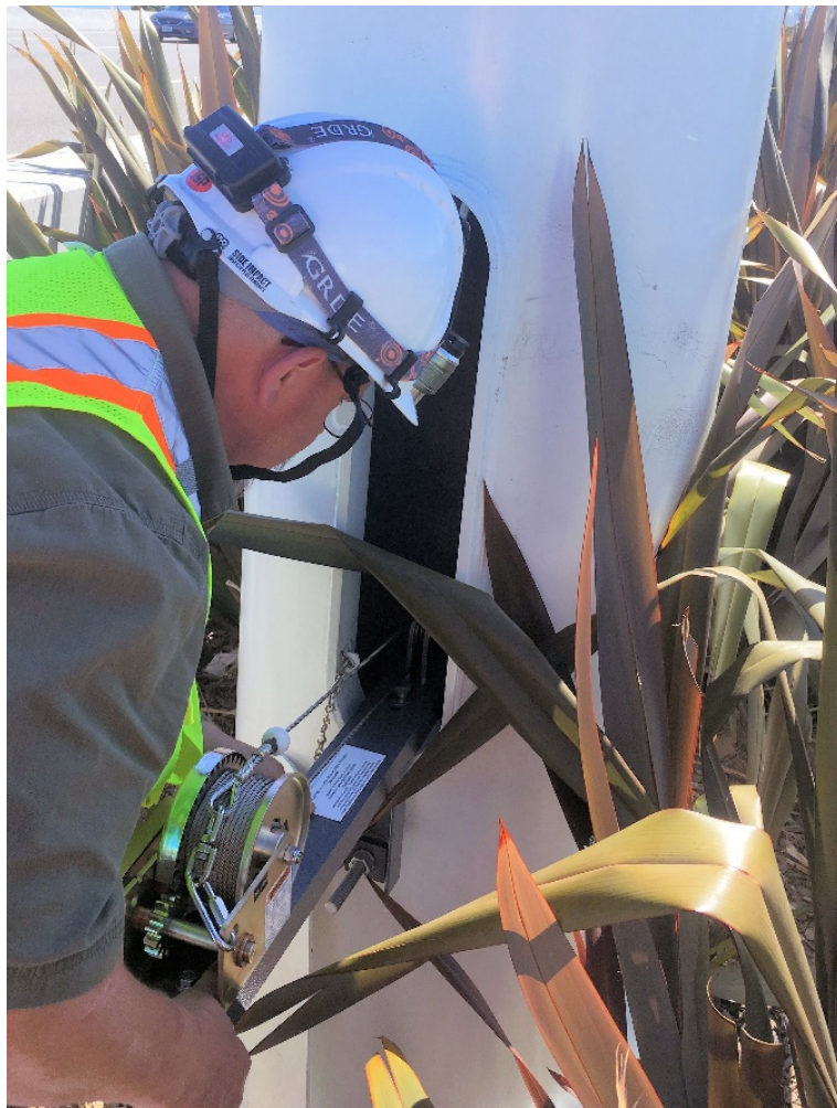
Figure 62. Attach Winch Tool
