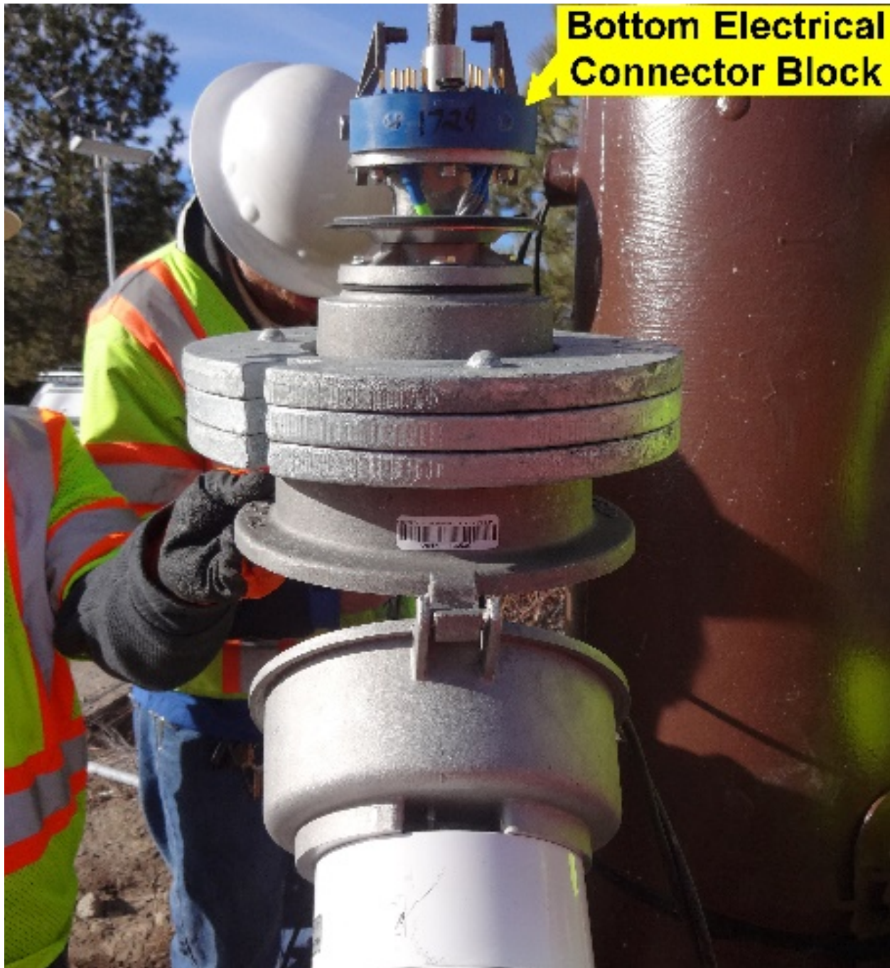
Figure 11. MG 2 E-Connector Installed
