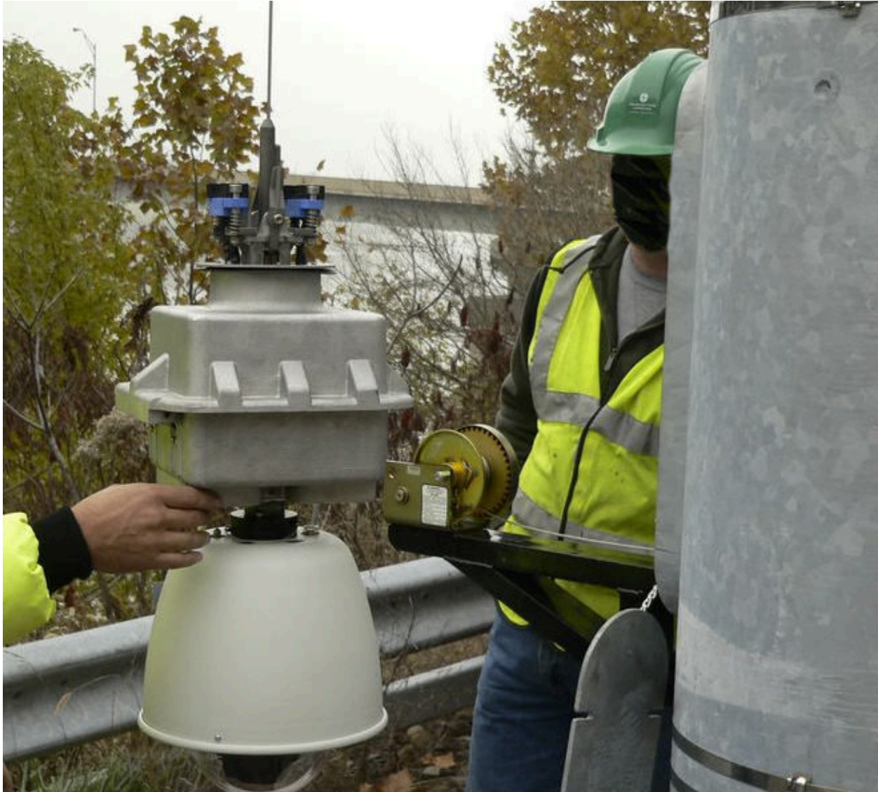
Figure 16. Camera Lowering Systems, Inc. Camera Pendant Lowered (Image courtesy of Camera Lowering Systems, Inc.)
