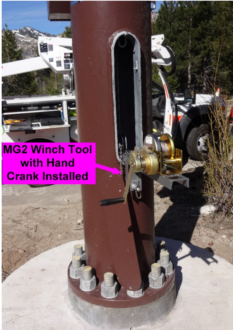
Figure 49. Meyers MG 2 Lowering Winch Tool
