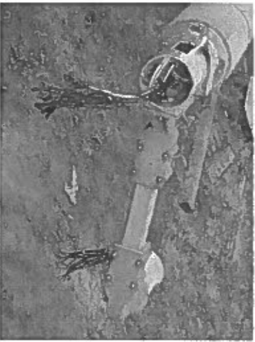
Unroll Composite Cable Hand over Hand to avoid Kinks
