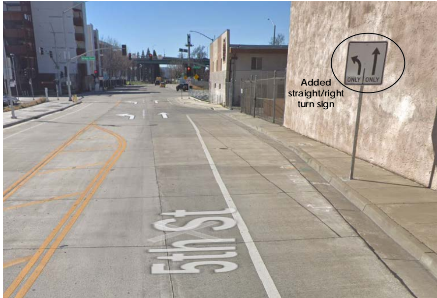
Figure 4.38: Caltrans' sign addition for southbound 5 th Street on the north side of the intersection at the South River Road exit ramp. Image courtesy of Google Street View.
