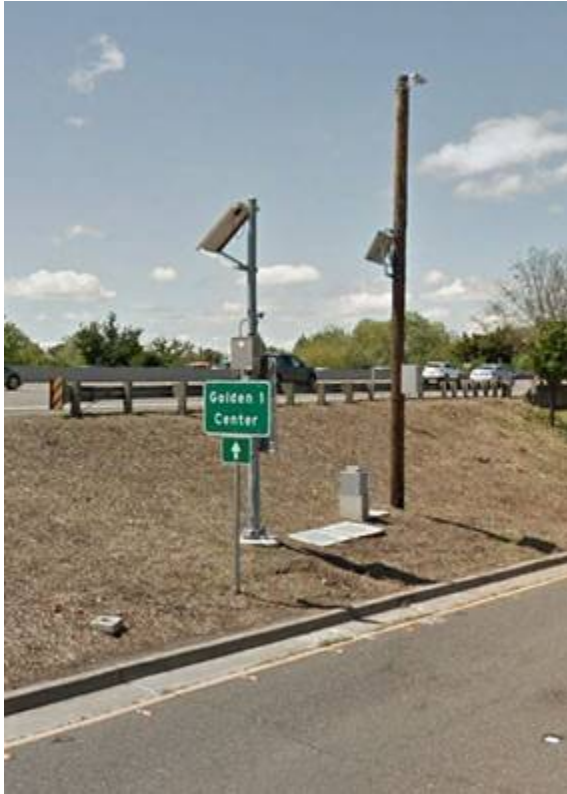
Figure 4.41: TAPCO radar sensor blocked by informational sign for the 16 th Street exit ramp system. The AHMCT VBSM can be seen behind the TAPCO system.
