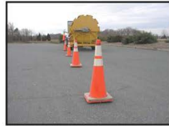
130 cones will cover 1 1/4 miles at 50' spacing or 2 1/2 miles at 100' spacing.
