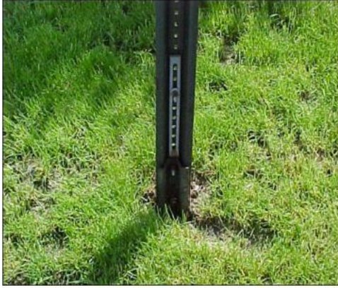
Figure E.12: Channel bar breakaway post. Image courtesy of PennDOT [19].
