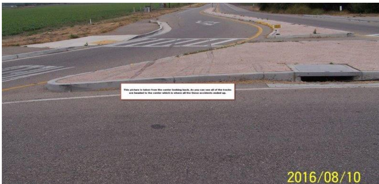
Figure A.9: This picture is taken from the roundabout center looking back. Tracks are headed to the center which is where all these accidents ended up. Skid marks indicate people speeding. If there was landscape in the splitter island, workers could have been hit during maintenance. Image courtesy of Caltrans.
