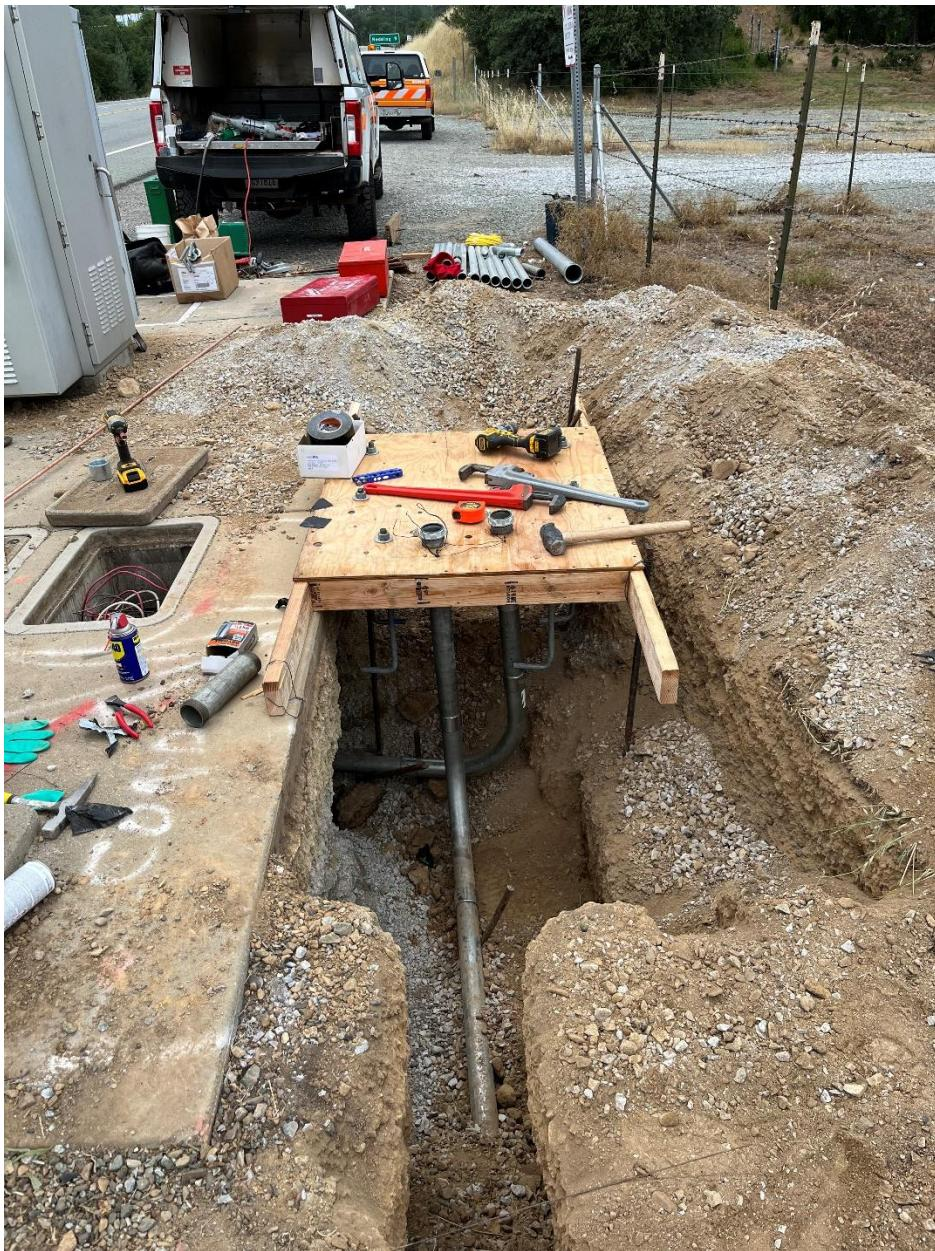
**Figure 5.2: Construction Photograph of the Foundation Form for the HyMax System**
