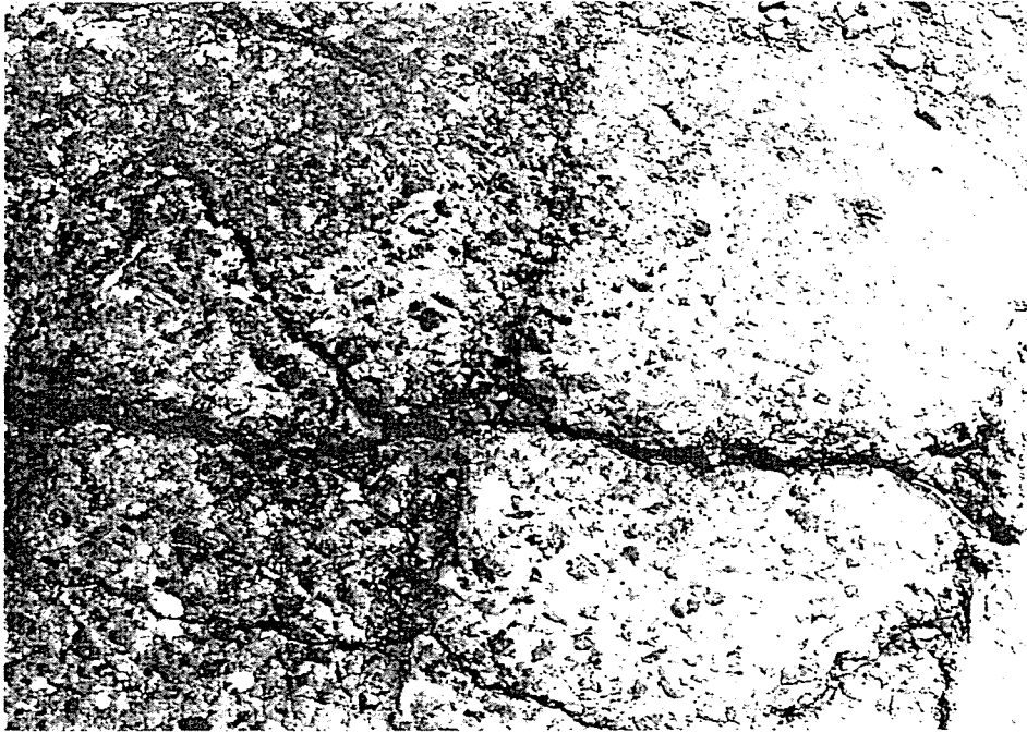
Photo 2.15 - "Before and After" - Cracks Cleaned with Compressed Air
