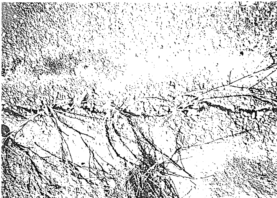
Photo 3.19 - Crack Area After Sandblasting
