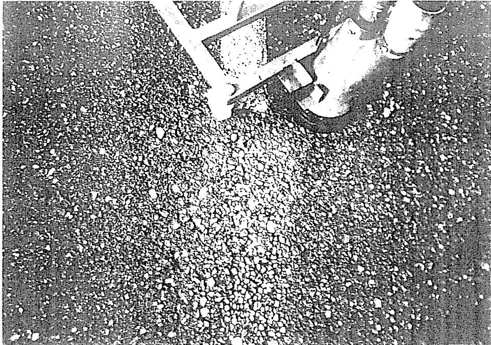
Photo 3.33 - Paint Stripe Removal Using the Vacuum Blast Method
