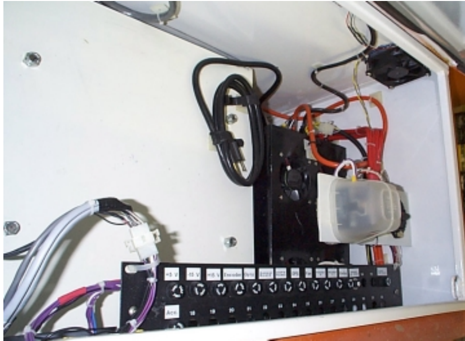
Figure 3-10: ASP Power Supply System
